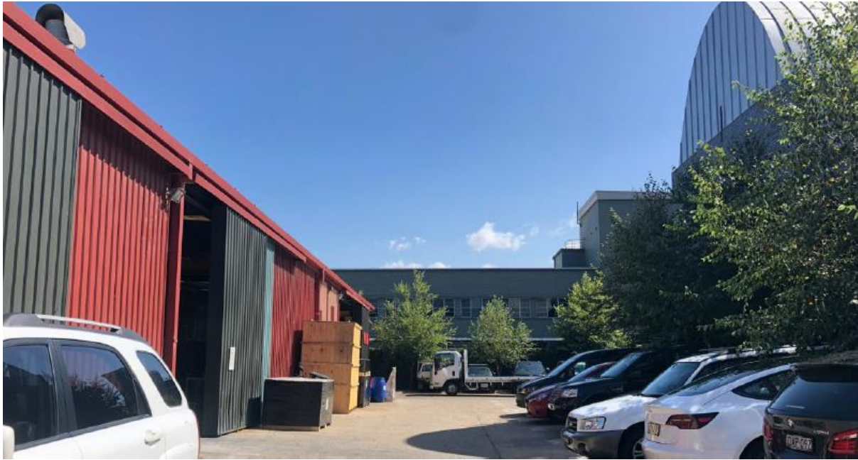
Figure 5: Existing driveway and parking area between Building 1 (right-hand side) and Building 2 (left-hand side) looking west
