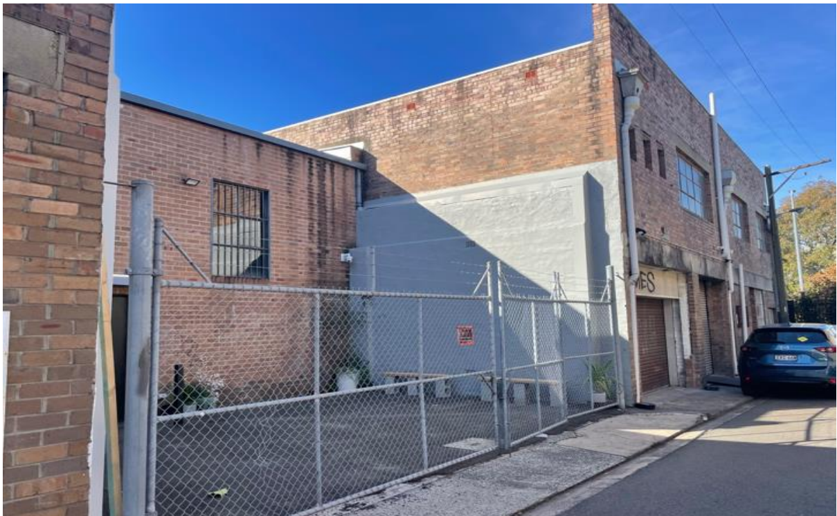
Figure 12: Adjoining development to the east of the site fronting Balaclava Lane
