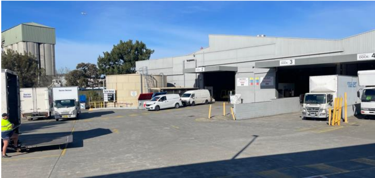
Figure 9: Development to the south of the site known as 30-32 Bowden Street which comprises a variety of uses including a warehouse and office building for Harvey Norman, an office premises, a commercial arts studio and fitness centre
