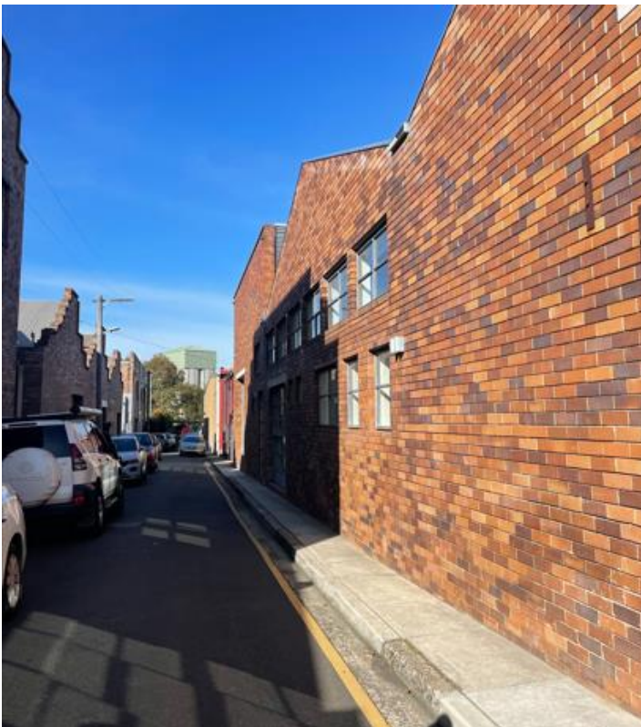
Figure 14: View looking south down Balaclava Lane, with Building 1 located on the right-hand side
