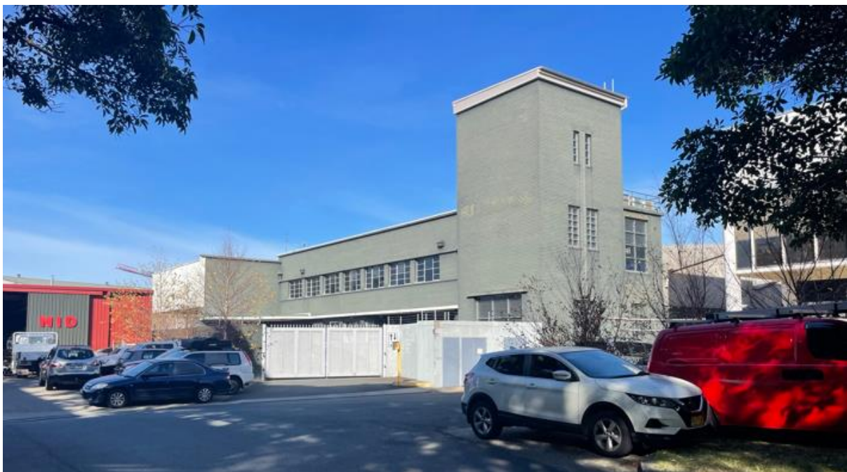
Figure 6: Development located to the west of the site known as 20 Stokes Avenue which is used as a premises by NSW Police and Bomb Disposal Unit as offices, training facilities, mechanical repairs and storage
